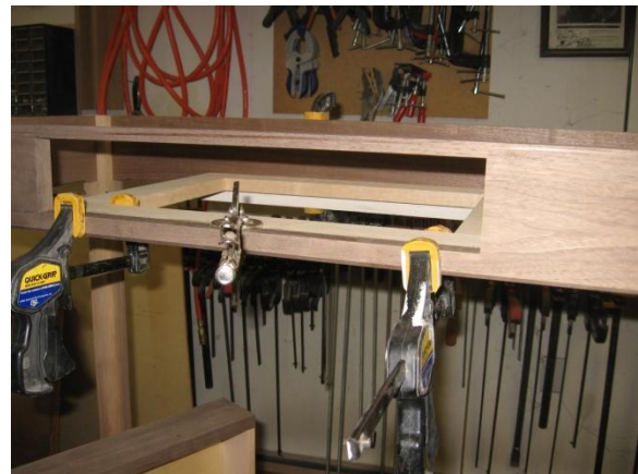
Figure 15 The frame being glued to the front apron flush with the bottom edge of the drawer opening.
