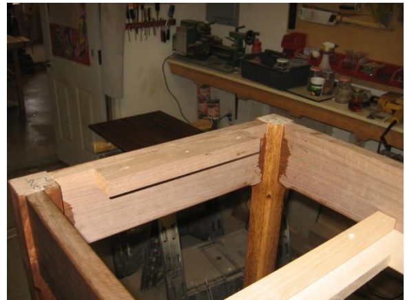
Figure 19 Attachment block for fastening table top to base allowing for expansion and contraction.
